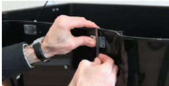
2. Using a 5/32" drill bit, steady the plate with one hand and carefully drill 1 hole. Install one 1/2" machine screw and nut and tighten slightly to stabilize the plate's location. Drill a 2<sup>nd</sup> hole and install a 2<sup>nd</sup> screw and nut. Complete drilling the remaining two holes. Remove plate, screws and nuts.
